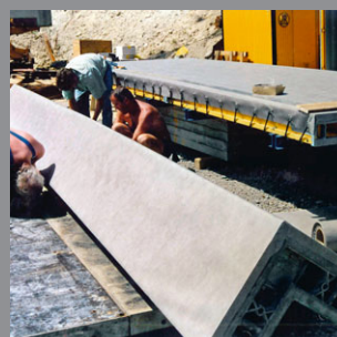
Drinking water reservoir, Schlüsselfeld (DE), 1992
