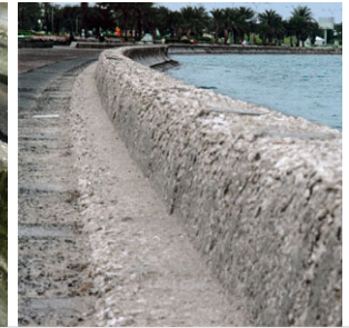
Results of salt crystallisation in a marine environment
