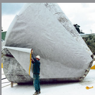
Wastewater treatment plant Munich (DE), 1990
