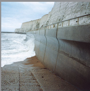
Seawall Brighton (UK), 1992
